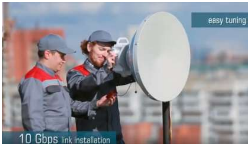
Fig. 27. Check RSL meter indication when running alignment procedure
