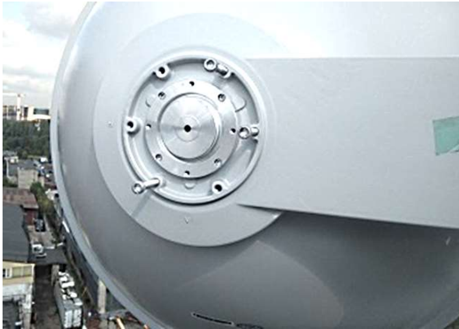
Fig. 44. Install 3 bolts on positions of "5, 15 and 35 minutes" on the antenna flange
