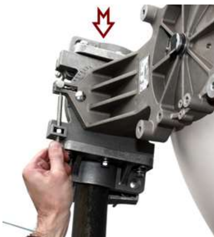
Fig. 16. It is more easy to put the antenna on top of the pipe than reassemble the mount to "hug" the pipe
