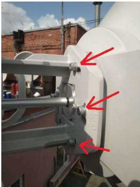
Fig. 45. Use 6 bolts to screw diplexer to antenna flange
