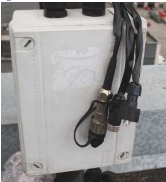
Fig. 12. Cross-connection box with power, UTP and fiber cables to transceiver
