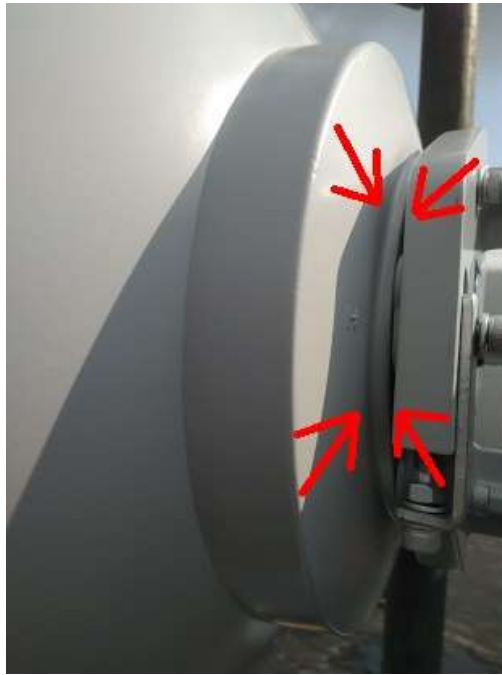
Fig. 46. Do not allow the appearance of an uneven gap between the antenna and the diplexer
