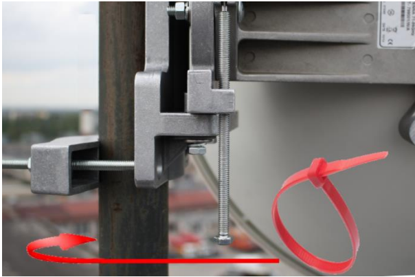
Fig. 17. A plastic tie strip tightening on the pipe stand will not allow the mount to slip down during installation procedure and thus prevents antenna from possible damage
