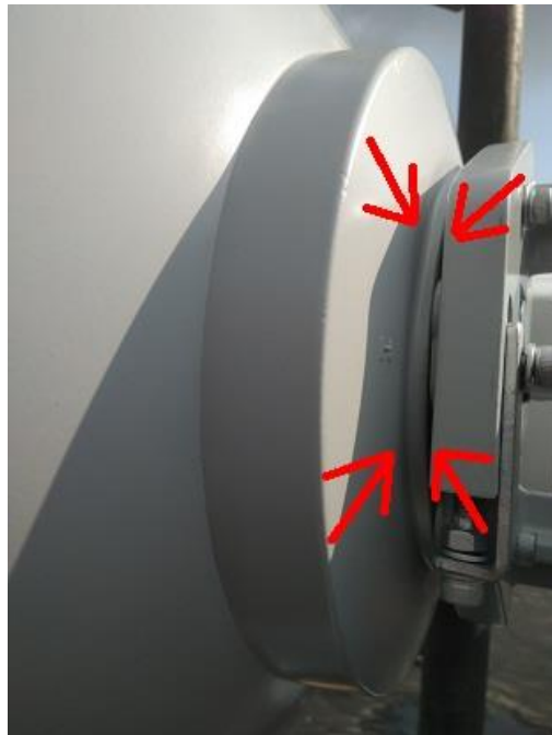
Fig. 42. Do not allow the appearance of an uneven gap between the antenna and the diplexer
