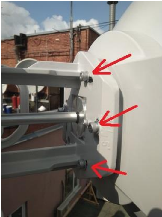
Fig. 43. Use 6 bolts to screw diplexer to antenna flange
