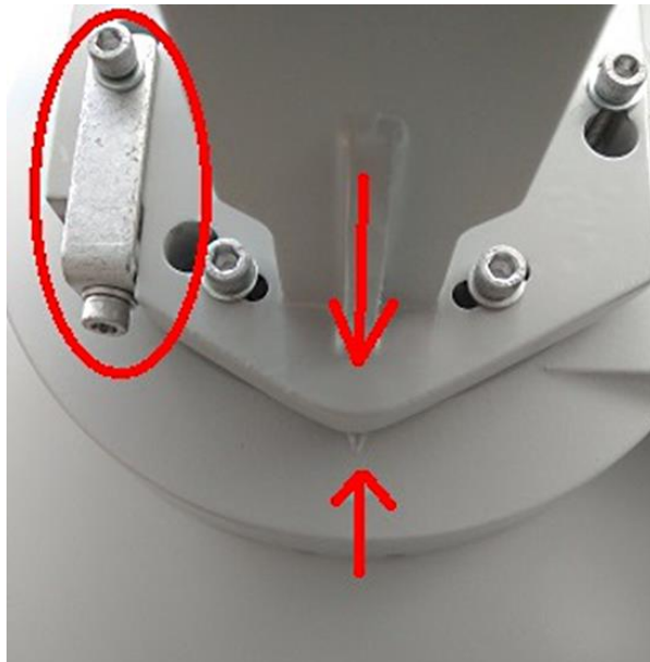
Fig. 44. Adjust the diplexer rotation using the element marked by red oval
