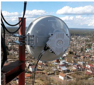
Fig. 9. Radio could be installed on vertical or horizontal pipe
