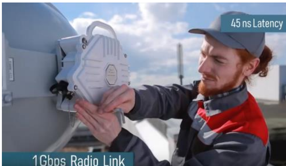
Fig. 1 PPC-1000-LL link at the point of installation
