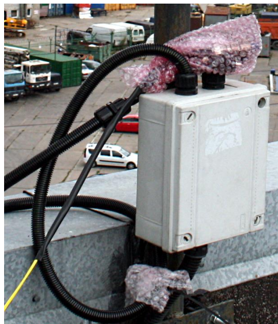
Fig. 12. Cross-connection box with power, UTP and fiber cables to transceiver
