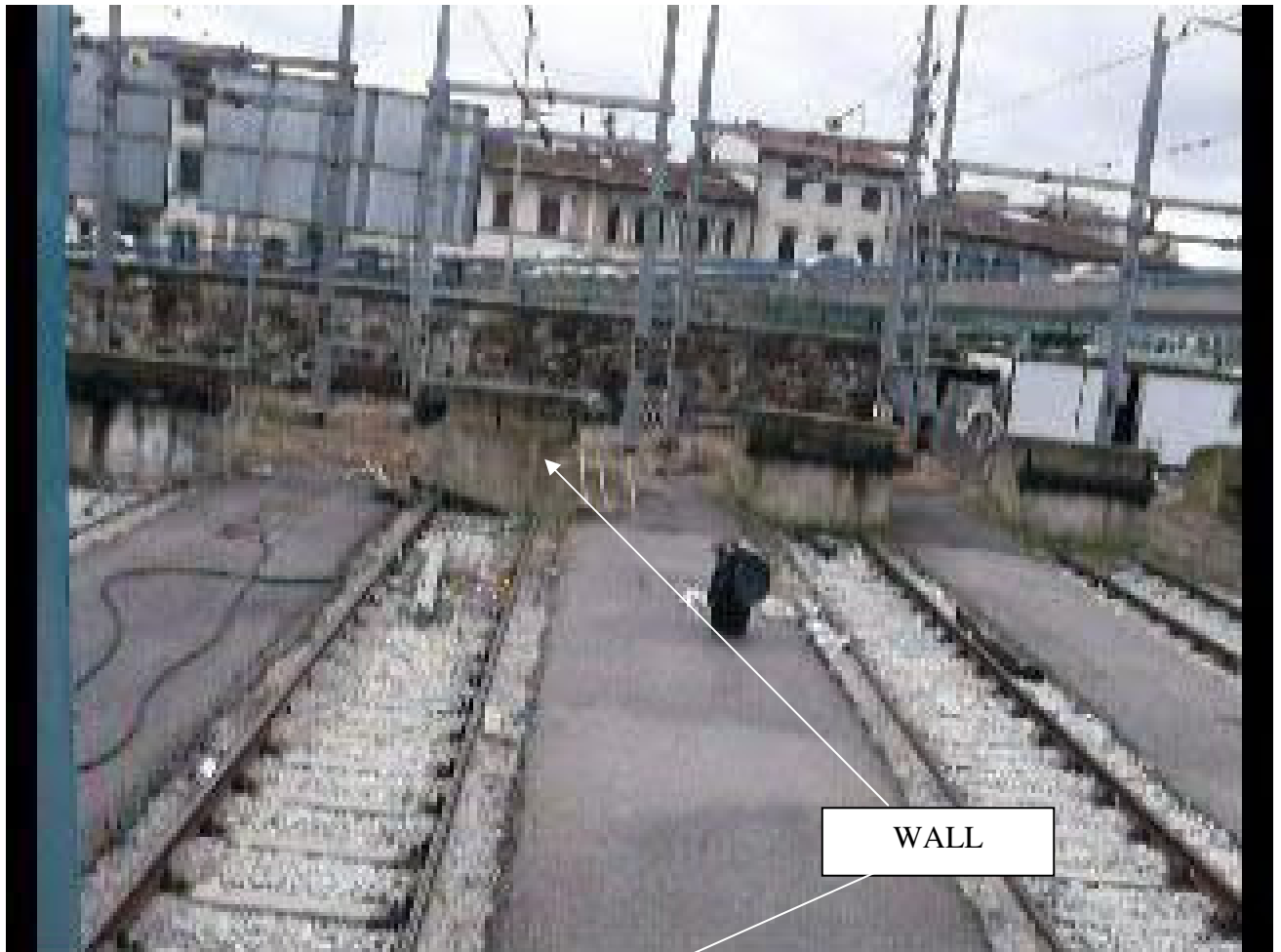
The wall at 24m.
