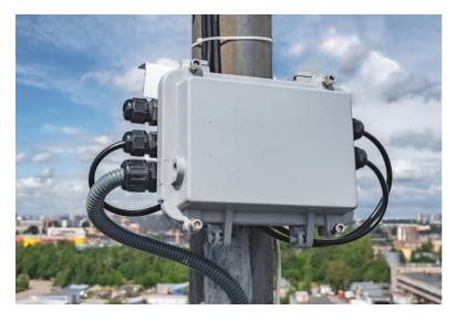
MESH network node routers (EDGE routers) are located in close proximity to radios and are used to manage routes, bandwidth, QOS, etc. Unlike classic network routers, they are less expensive, compact, cooler and use less electricity.
