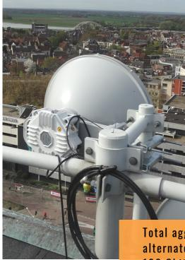
10Gbps 70-80GHz E-band radio links are ideal for the deployment of wireless mesh network at the city scale.
